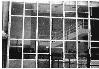
This is not an open stair—don't be fooled.
